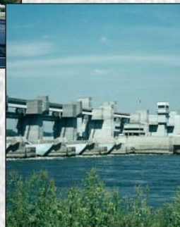
Lock and Dam
